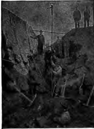
Fig. 118. Hammer Drill Drilling 15 ft. Holes.
